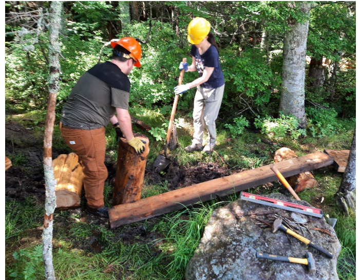
Volunteers work together to dismantle old deteriorated bog bridges
