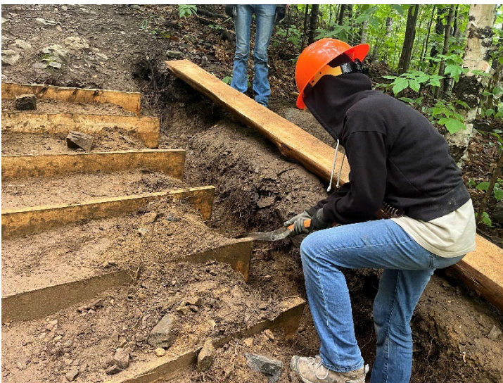
Left: Crew member makes adjustments to the steps before setting in the side rail
