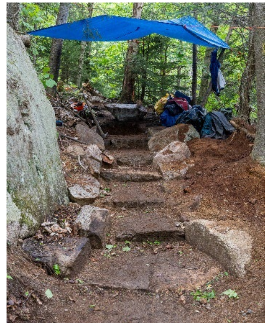
Steps set with scree, rocks lining the steps to ensure hikers walk on the durable steps
