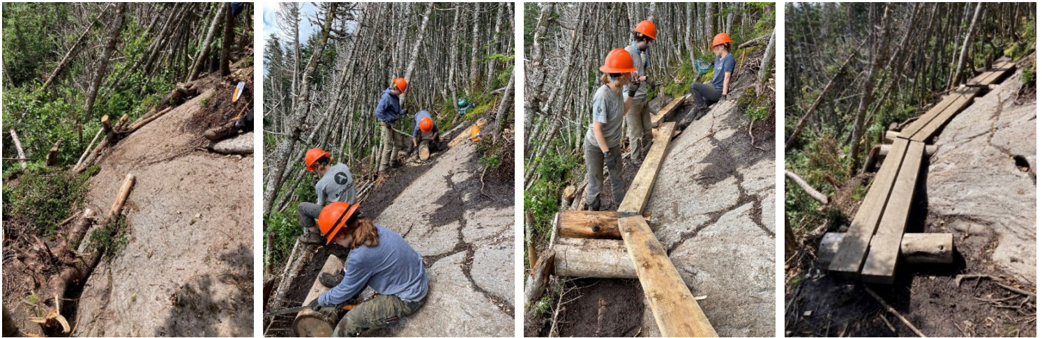
Above: The progression of building up the bio mass retention wall, cutting base logs to fit the area, laying out bog bridges, and the finished product.
