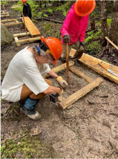
Painstaking attention to detail resulted in sturdy, level bog walks
