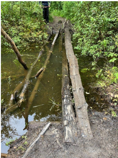
The old bog bridge was clearly in need of replacement
