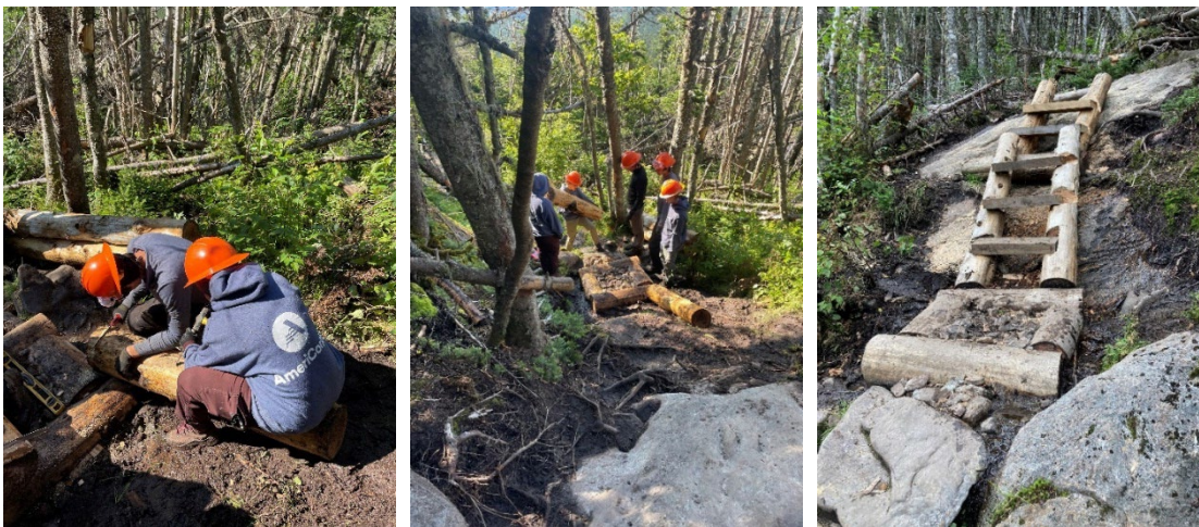
Below: Crew members cut logs to size, and then place rails for the ladder. Notches were then cut for the steps, and steps were placed
