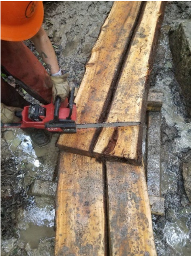
Crew Leader Sophia Weisman-Rowell uses a chainsaw to cut the cedar planks so that they line up neatly
