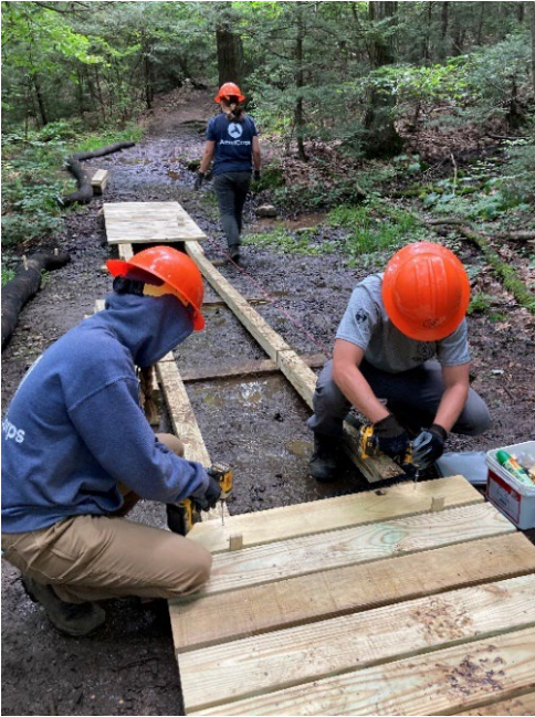
Crew members fasten decking one of the boardwalk
