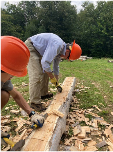
Volunteers used hand tools to hew the top of each cedar log to create a flat walking surface.
