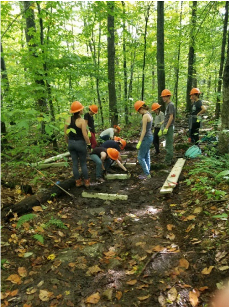
Volunteers lay out base logs for the bog bridges
