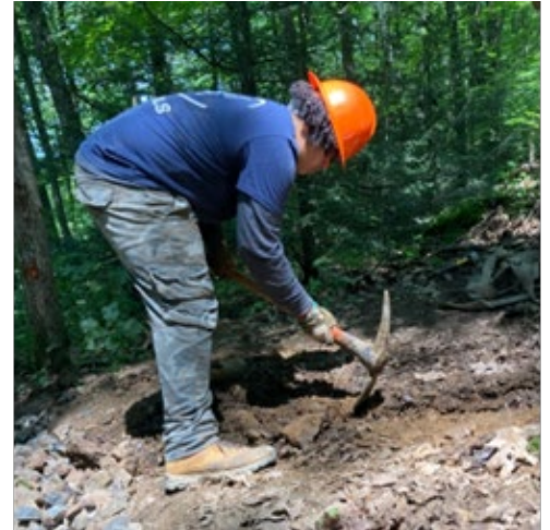
A crew member digging where a rock water bar will be built across the trail
