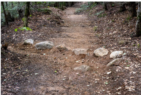
A rock waterbar placed at the top of a stretch of check steps, to help water drain off of the trail
