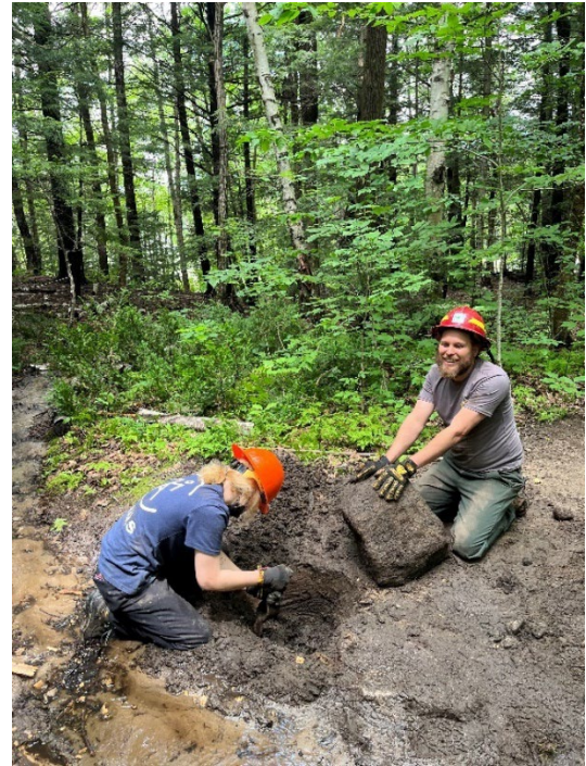
James and Ariya set a rock for a water bar
