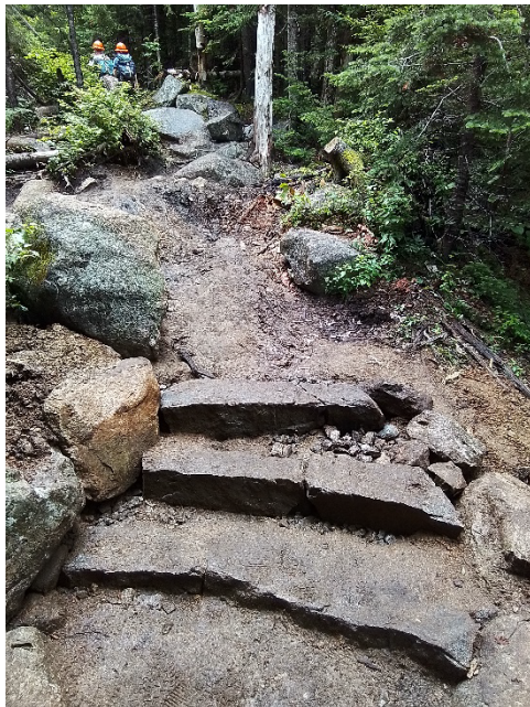
Two rocks are set next to each other to create a wider walkway
