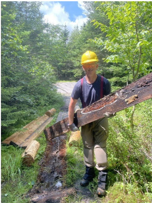
Removing old bog bridges and making way for new
